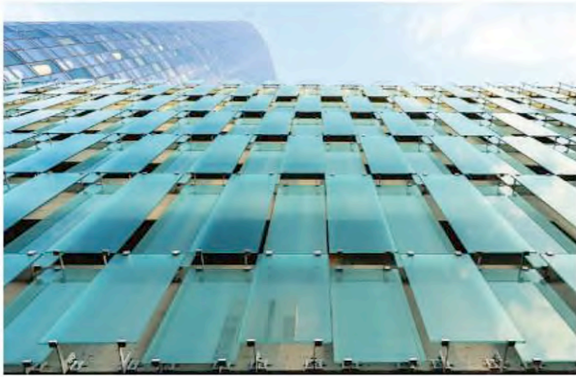
The north elevation of the parking garage on 727 West Madison in Chicago with staggered 'in-out' glass panel layout for natural ventilation.
