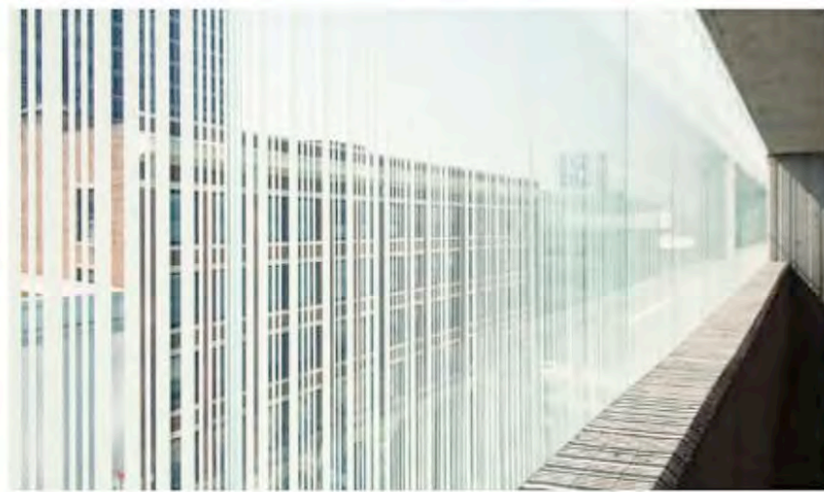
The custom pattern-fritted glass provides solar shading, while maintaining occupants' visibility to the outside.
